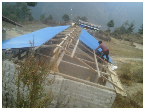
Community-led construction of Shree Shanti Primary School in Lapu Village
