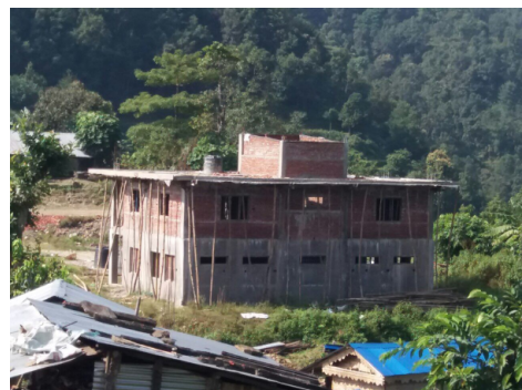
Reconstruction of Shree Himalaya High (Secondary) School in Sourpanni Village
